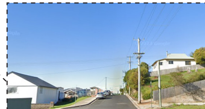
STEEP TOPOGRAPHY TO SOUTH END OF SITE INTERFACE WITH KING EDWARD ST PROVIDES OPPORTUNITY FOR INCREASED HEIGHT OF DEVELOPMENT TO TIE IN WITH CONTEXT.
