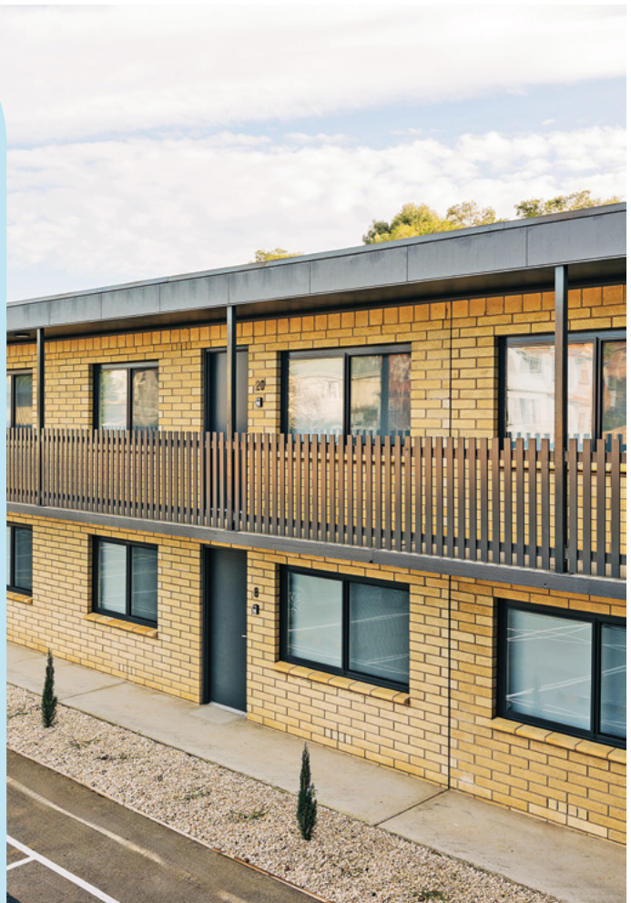
Key worker accommodation in Punchbowl | Photo Adam Gibson
