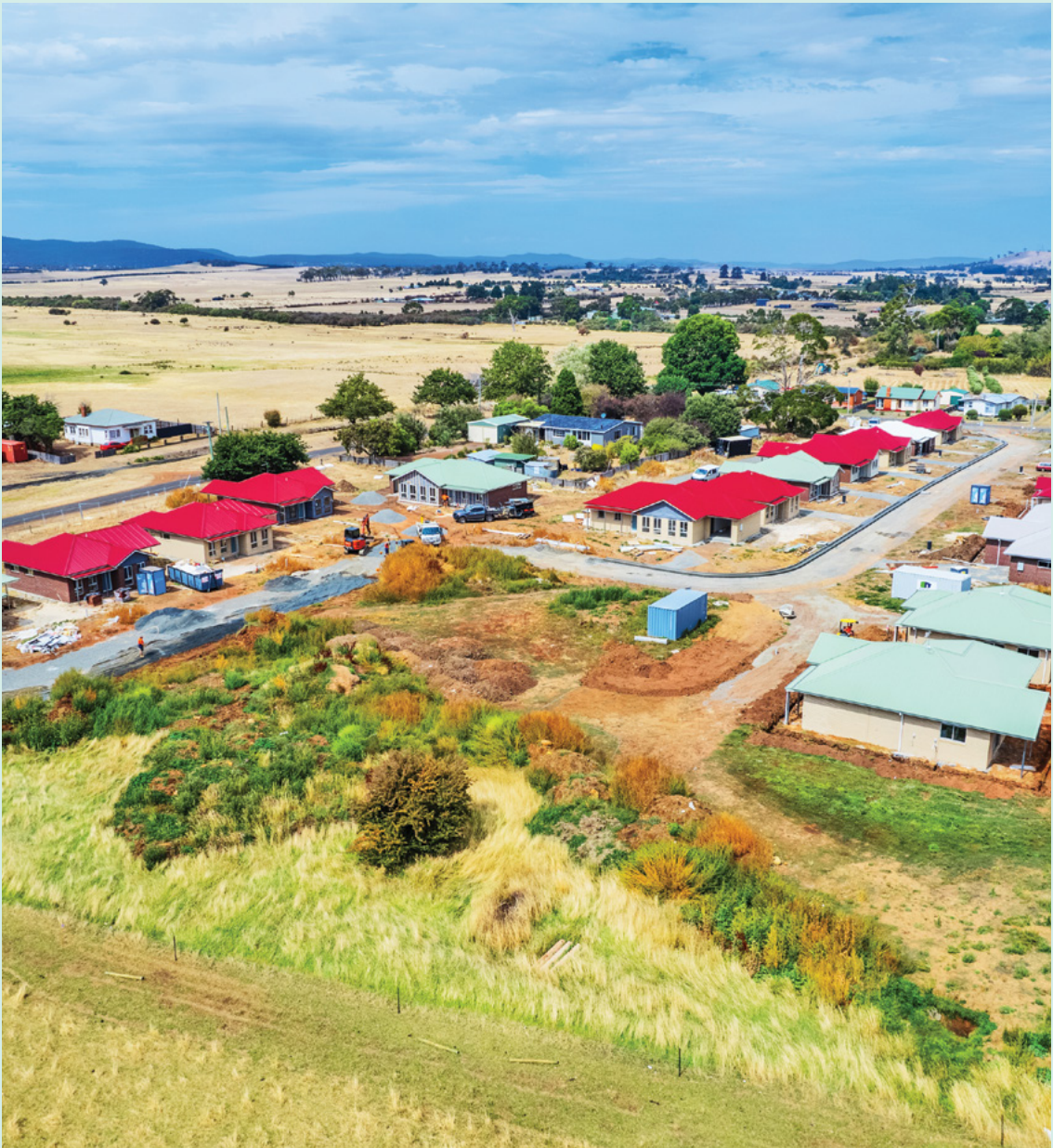
High Street development | Photo primeperspectives.com.au
